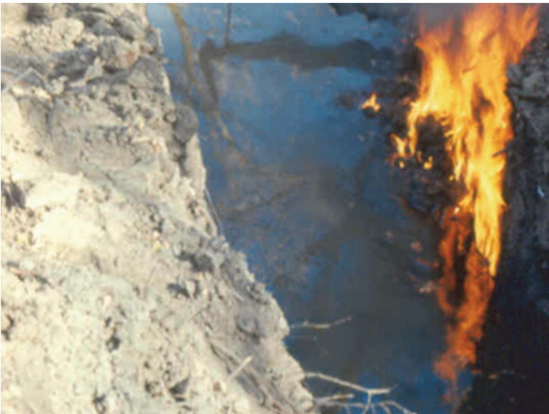
ISB of Oil Seeping into a Trench
