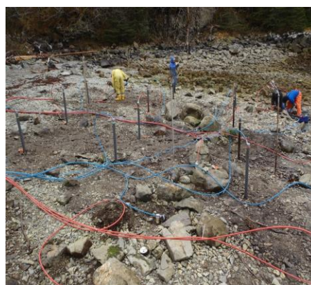
Figure 10: Injection wells for bioremediation of a beach in Prince William Sound, Alaska. The solution and pumps were placed landward of the beach.
