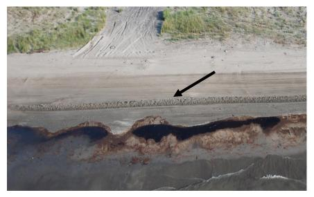
Aerial views of low (1-m) sand ridge being constructed by a road grader above the swash line as oil washes ashore.
