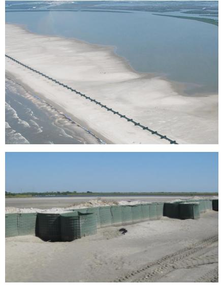
Armored baskets placed along the highest elevation on a long, low sand barrier.
