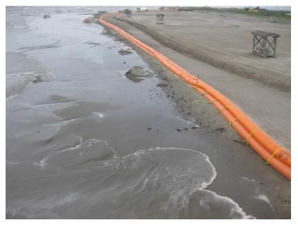
Water-ballasted boom anchored to form a barrier at the high water level. Note the low sand ridge on the landward side of the boom.
