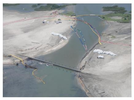
Solid sheet pile barrier under construction across a shallow channel. In the ground view at left, note oil in the lower half of the image. Hard booms, Super Sacks, and snare booms were deployed prior to completion of bulkhead construction.
