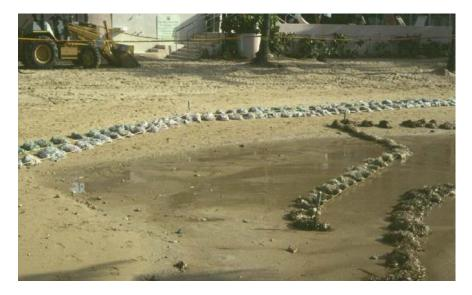
Snare boom placed in parallel in the upper intertidal zone to collect oil as it is washed ashore on a rising tide (T/B *Morris J. Berman* response, Puerto Rico).
