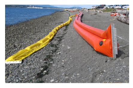
Conventional solid floatation boom and water-ballasted ("shore-seal") boom deployed at the high tide water level during an exercise (Port Angeles, WA).
