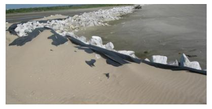
Geotextile barrier held in place by imported rubble across a low section of a barrier beach.
