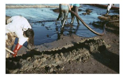
Trench being dug at the high water line to collect oil as it washes ashore on a rising tide (T/V *Estrella Pampeana* response, Argentina).
